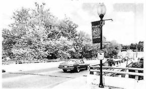
and used until the middle of the 1930's. In 1936 the present bridge was built of concrete and steel, which sits on two abutments and two center piers above the East Fork of the Little Miami river. At the time of completion it was thought to be a most beautiful bridge which should never need replacing.
